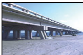
St. Luis Pass Bridge, TX
